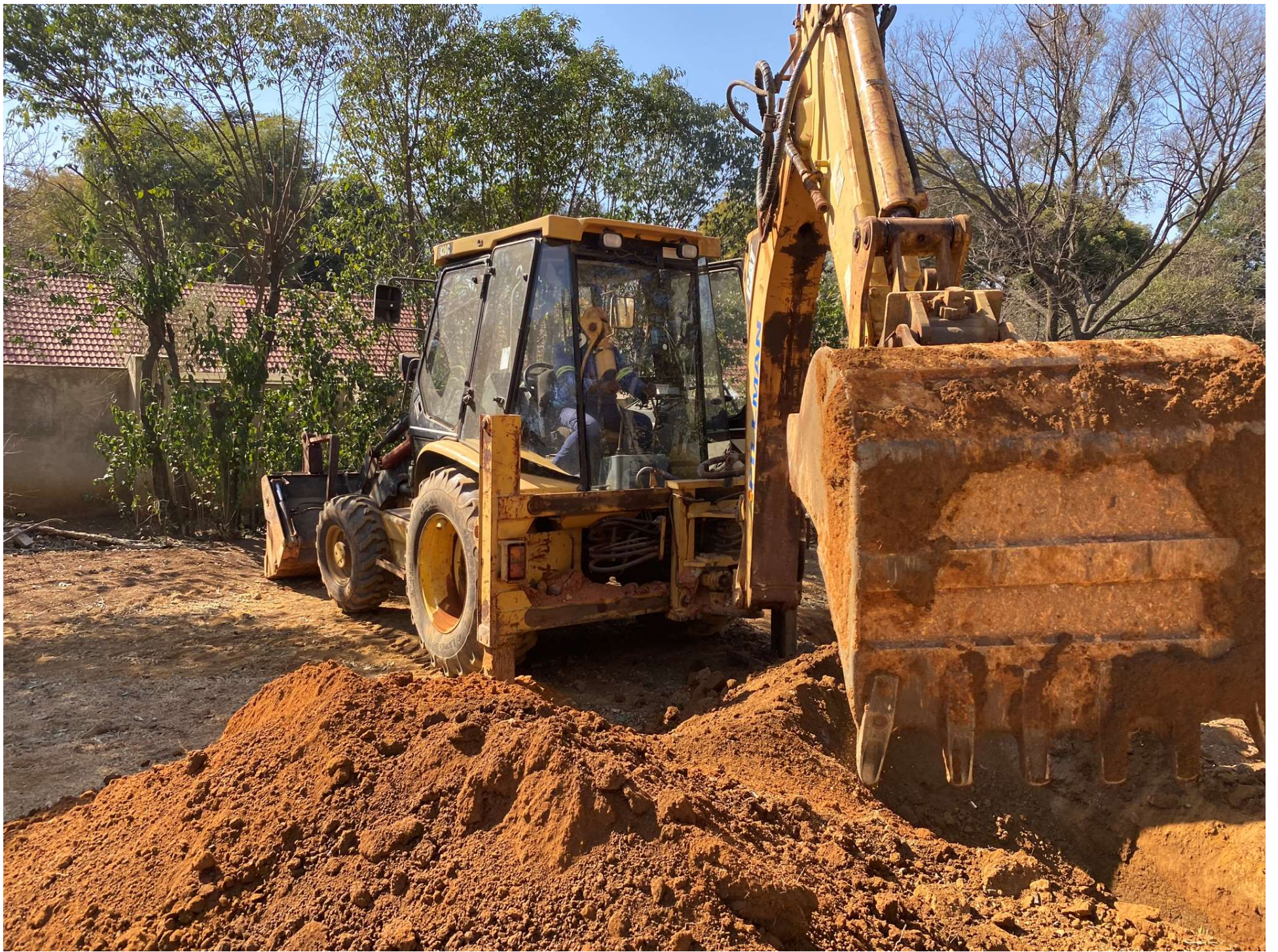
Digging of test holes
